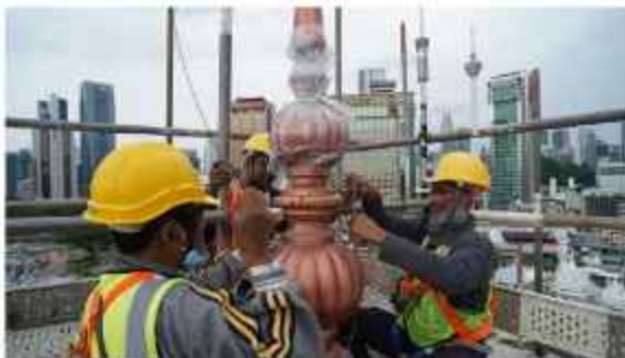
Pemasangan tunjuk langit baharu di tapak. The new finial was installed on site.
