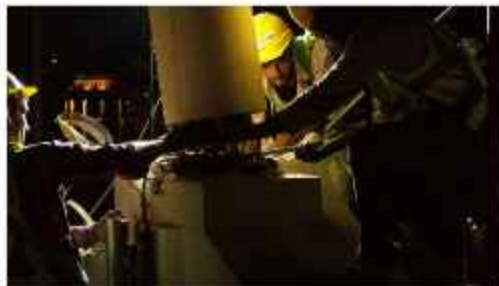
Pemastangan tunjuk langit baharu di tapak. Installation of the new finial on site.
