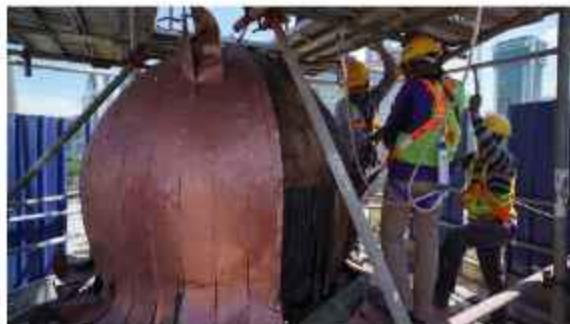
Kepingan kemasan kubah sedia ada direkod dengan teliti. The existing dome cladding sheets were carefully documented.
