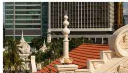
Tunjuk langit dipasang semula di bahagian parapet. The finial was reinstated on the parapet.
