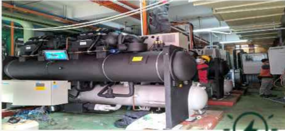
Retrofitting of Chiller with Magnetic Chiller
