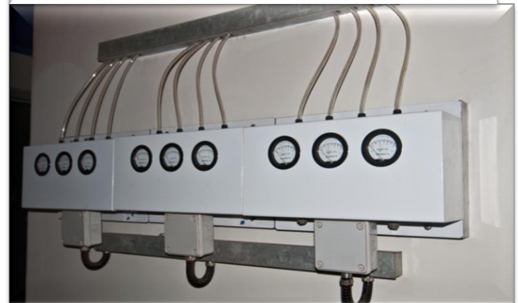
Pressure Differential Gauges
