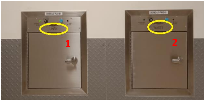
Full Vacuum Load Stations Linen waste collection, and General waste collection
